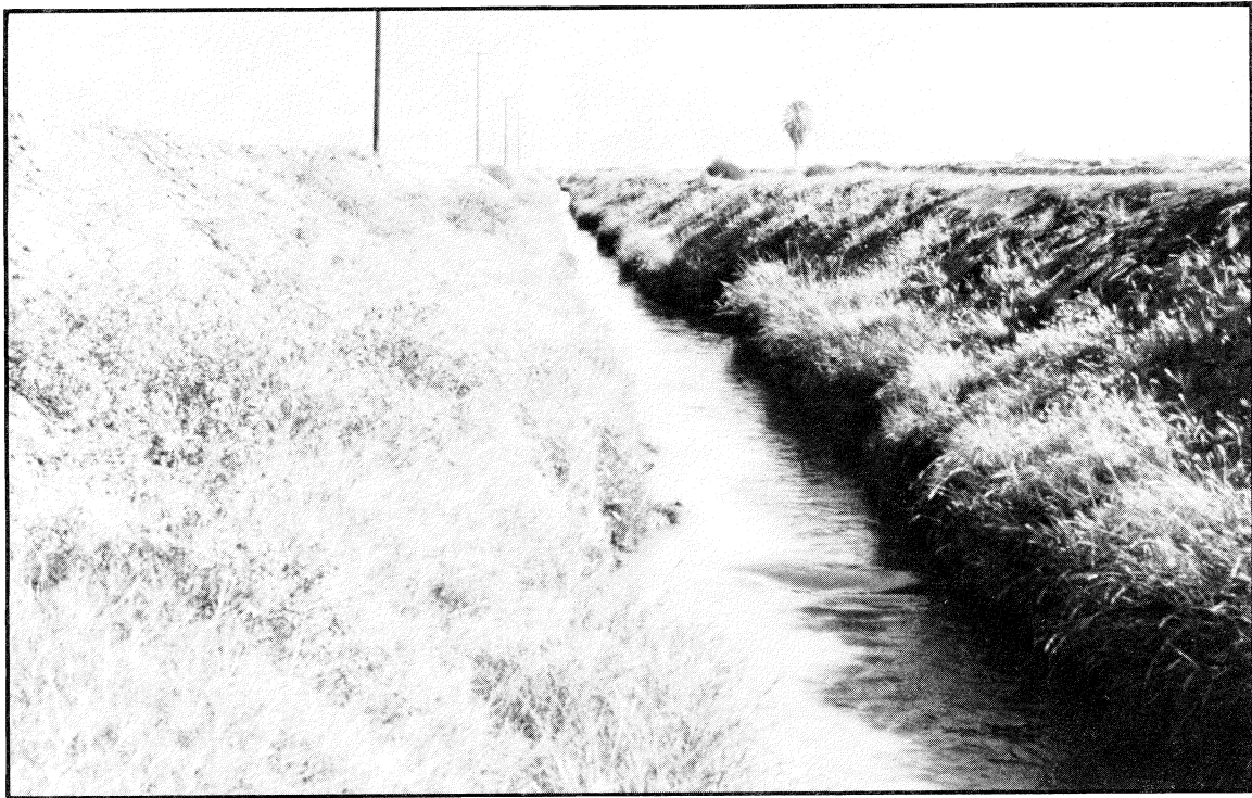
Collector ditch for drainage water from irrigated fields.
