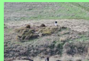
Fig. 2. Photo taken after trenching upslope and installing PVC standpipe (near center) for water collection.
